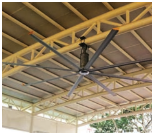
3 High-Volume Low Velocity Fan at Blk 23A Chai Chee Multi-Purpose Hall
