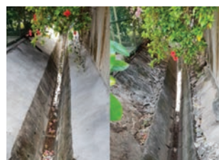
9 Clearing of Overgrown Vegetation and Crack Repair at Drainage between 47A and 49 Dunbar Walk
