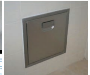
Replacement of refuse chute hopper
